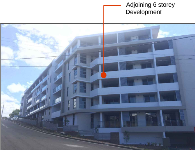
View of 20.5m height development at corner of Cook street and Henry street
